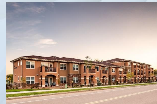
Mirasol Senior Facility
